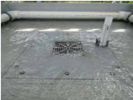
Weir Flow – 2.0 L/s (20mm)
