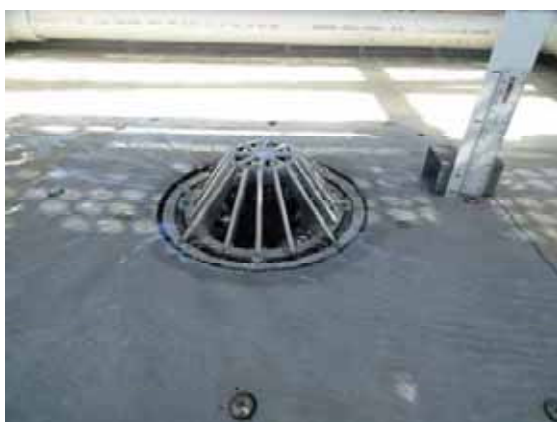
Weir Flow – 3 L/s (12mm)
